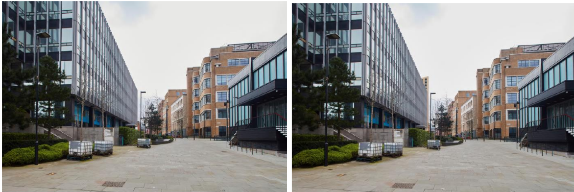
View 4 Dantzic Street/ Miller Street Baseline View 4 Dantzic Street/ Miller Street Proposed
