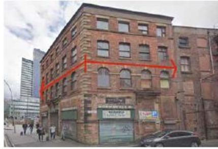
Extent of Facade to be retained
